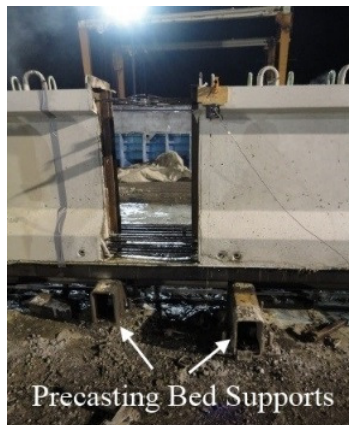
PPCB ends over the bed supports
